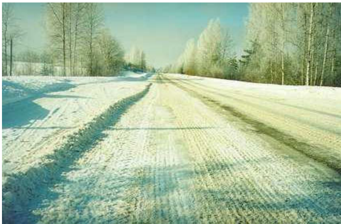
Figure 6 Wrinkled surface of compacted snow class B
