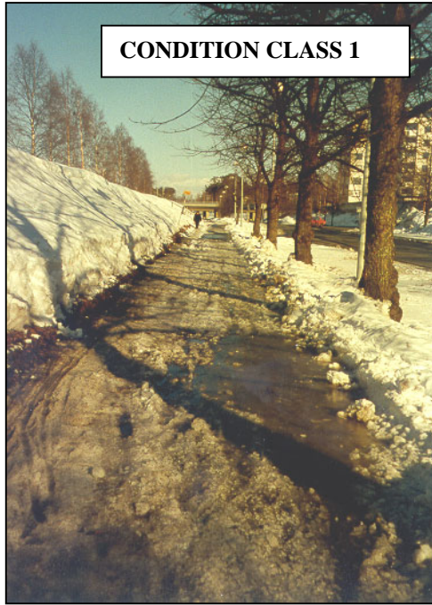
Figure 11. Water coming from snow melted by the sun refreezes on the route at night.
