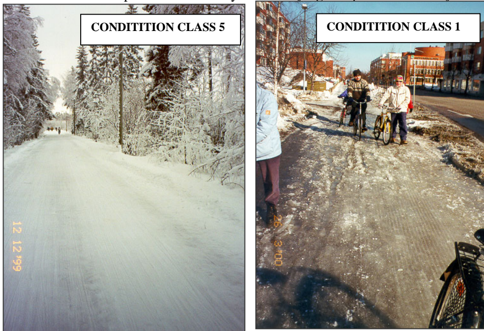
Figure 5. A cycle track maintained in an exemplary manner. Figure 6. A cycle track in an exceptionally bad condition.
