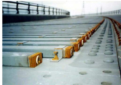
**Fig. 22 Steel pipes full of PCM**
