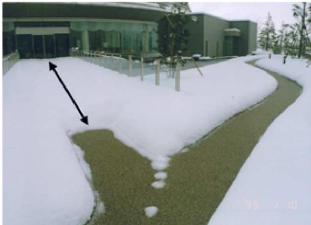
**Fig.7** Effect of thermal resistance between circulating water and road surface
