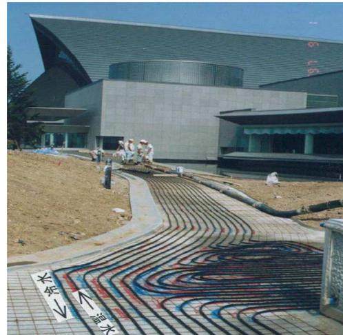
**Fig. 14 Works of dissipation pipes**
