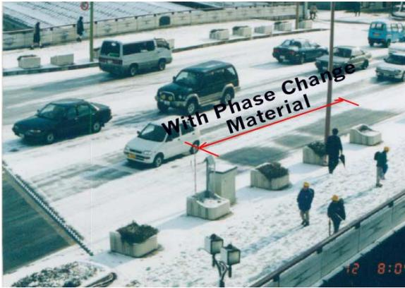
**Fig.25 Snow melting condition on steel deck with and without PCM**
