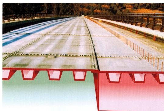
Fig.20 Frost condition on steel deck bridge
