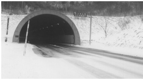
Photo 2 Snow-melting at the Koriyama-side entrance
