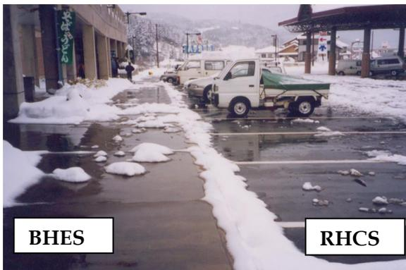
**Photo. 3** Snow melting condition of pavement connected to RHCS and BHES (Jan. 21, 2000)
