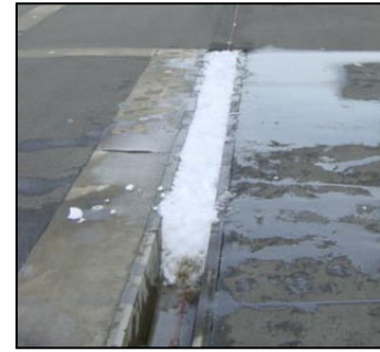
Photograph 5-1-4 Signal Wire Covered with Snow
