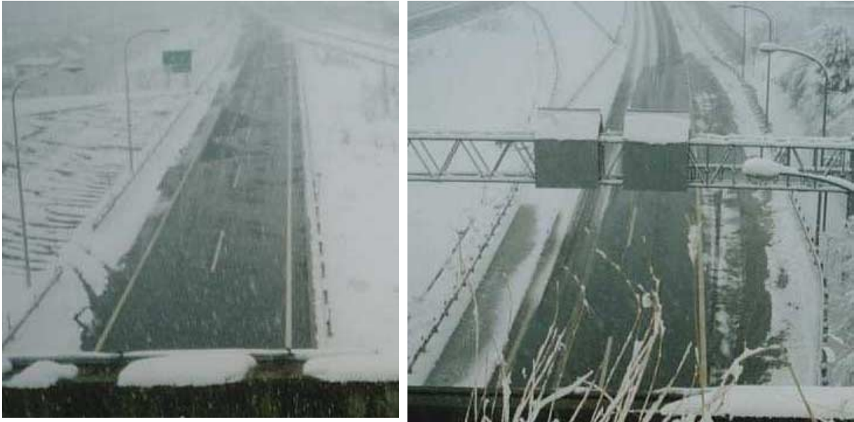
Nou TN Ups side pithead Porous asphalt pavement
