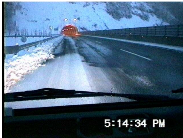
Onibushi TN Kanayama TN Photograph 3 snow melt situation by snow melting equipment with water sprinkling
