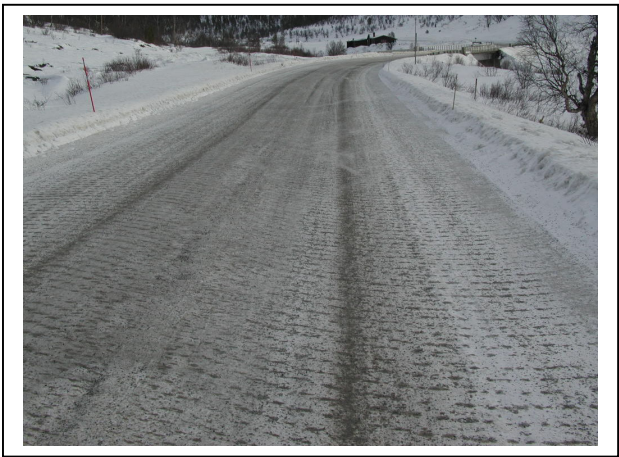
FIGURE 4 Typical Pattern on the Road using Warm Wetted Sand and a Spinner.
