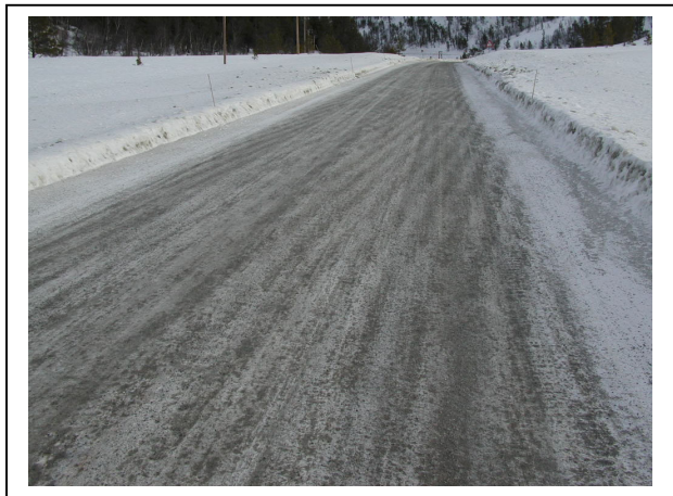
FIGURE 3 Typical Pattern on the Road using Warm Wetted Wand and a Roller Distributor.
