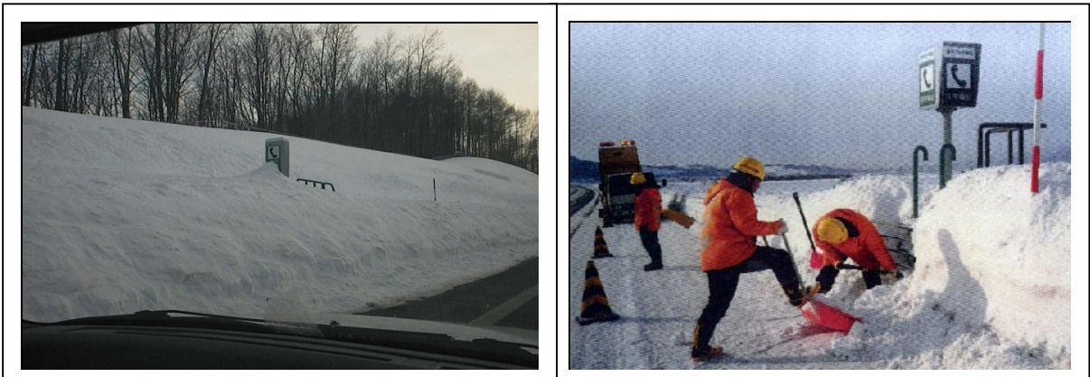
Fig. 8 Snow around an emergency telephone and manual removal of snow
