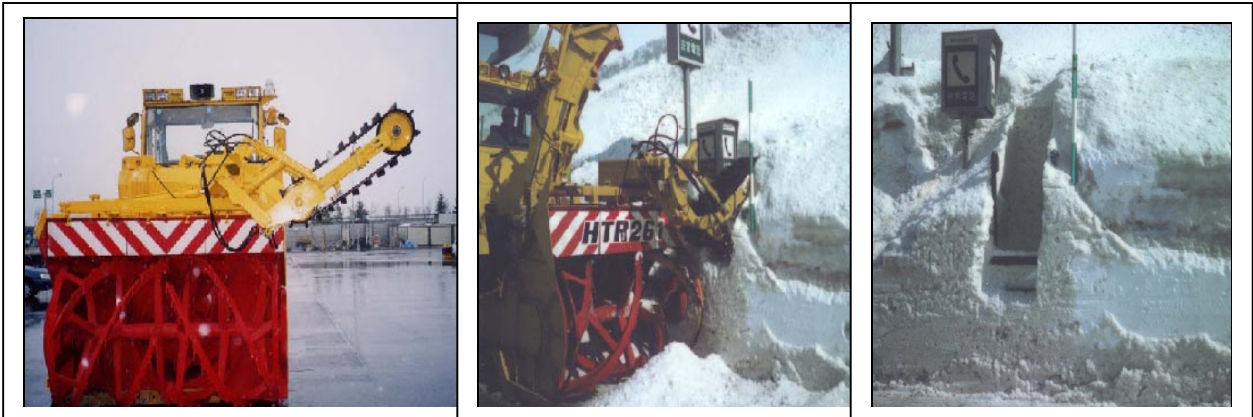
Fig. 9 Snow removal around an emergency telephone using a snow-removal machine
