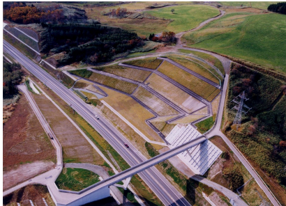
Figure 3 Slope failure site (After reconstruction)
