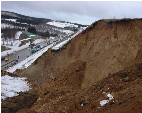
Figure 19 Slope failure site and drainage area
