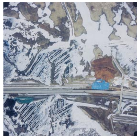
Figure 1 Kuromatsunai area and slope failure site (April 15, 1999)
