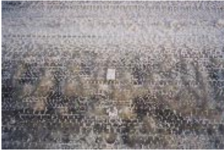
Compacted Snow on the Porous Asphalt
