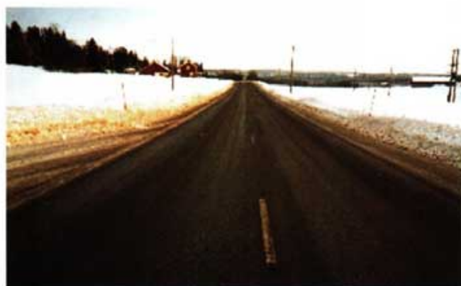
Figure 9 The most common road condition in the winter is bare road
