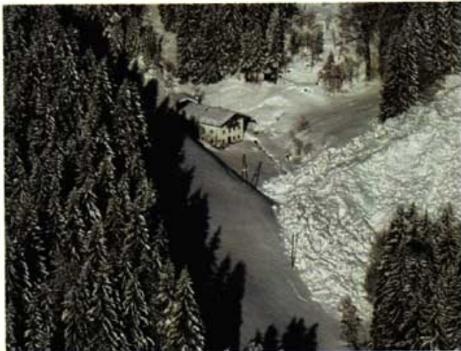
An experienced farmer has built his farmhouse near Unken, Salzburg on a protected site. Unfortunately the access to his house is not safe. Locally large quantities of fresh snow led to overload and to a big avalanche.
