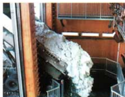
Heat sources of snow-flowing tanks 1) processed sewage that already carries heat to melt snow, and 2) residual heat from incineration plants, etc.
